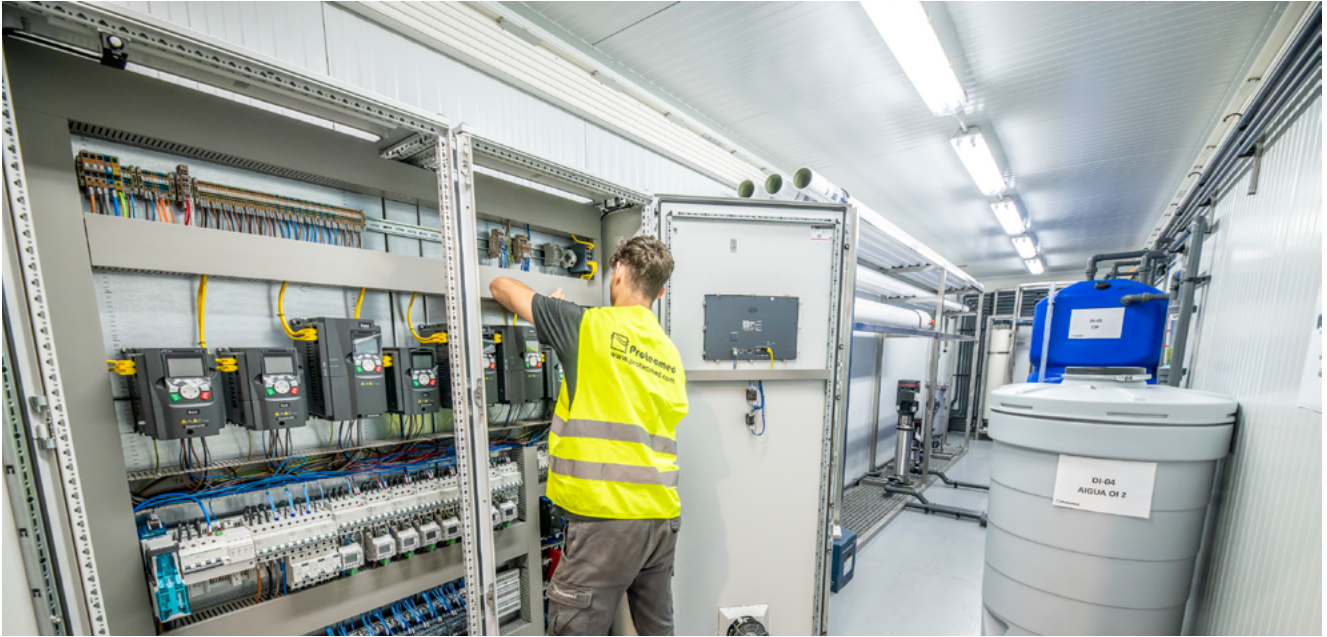
An operative sets up the pilot plant for the purification of water from the Wastewater Treatment Plant in Roses. The plant incorporates six different processes to guarantee the elimination of any potential contaminants and pathogenic agents.
